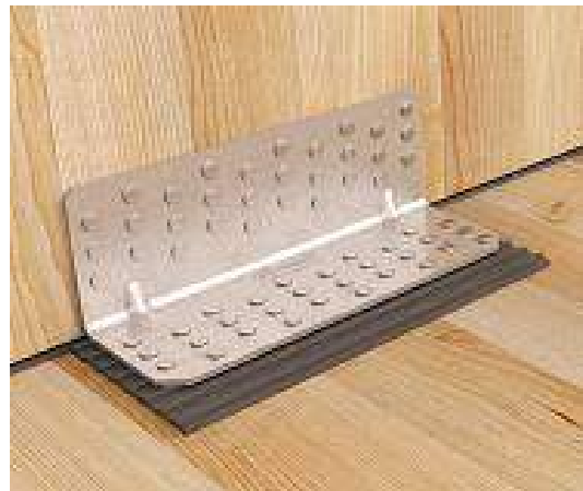
Figure B. 19 Typical installation TITAN Silent
