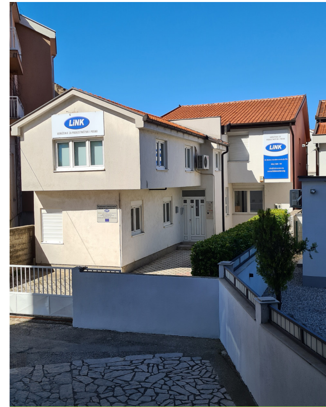
LiNK's premises in Mostar (Photo by LiNK Mostar)
